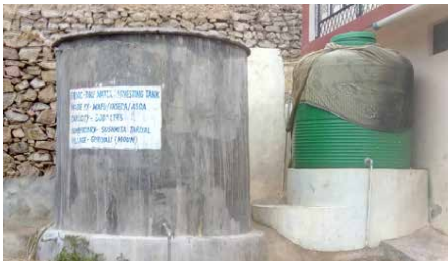
Rain water harvesting tank
